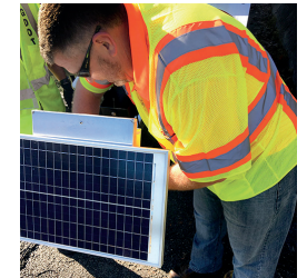
Connect batteries and test components before erecting the pole system.
